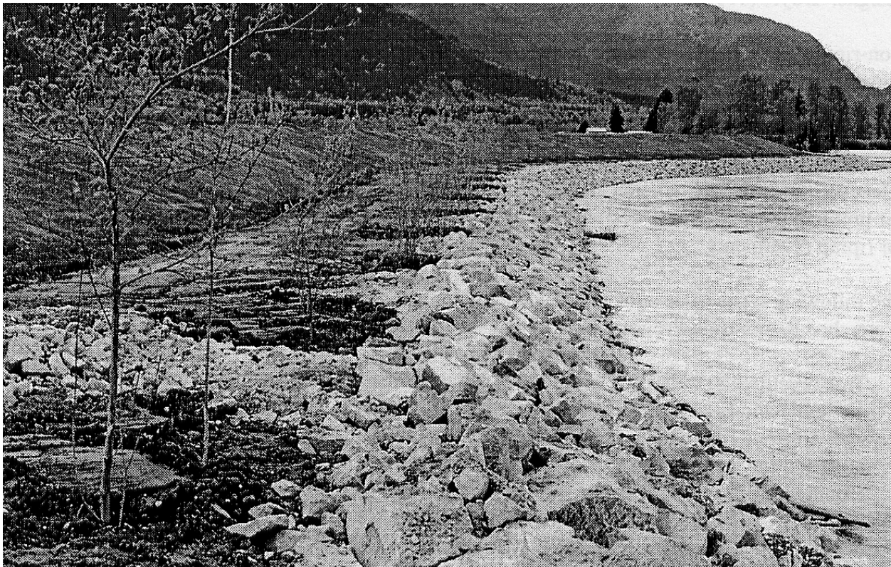
Figure 5-1: Planted Bench in Revetment along Nicomen Island, Fraser River
