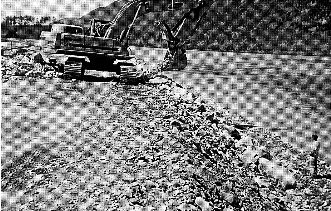
Figure 4-1: Placing Rock Riprap Over a Filter Layer on a 2H:1V Slope
