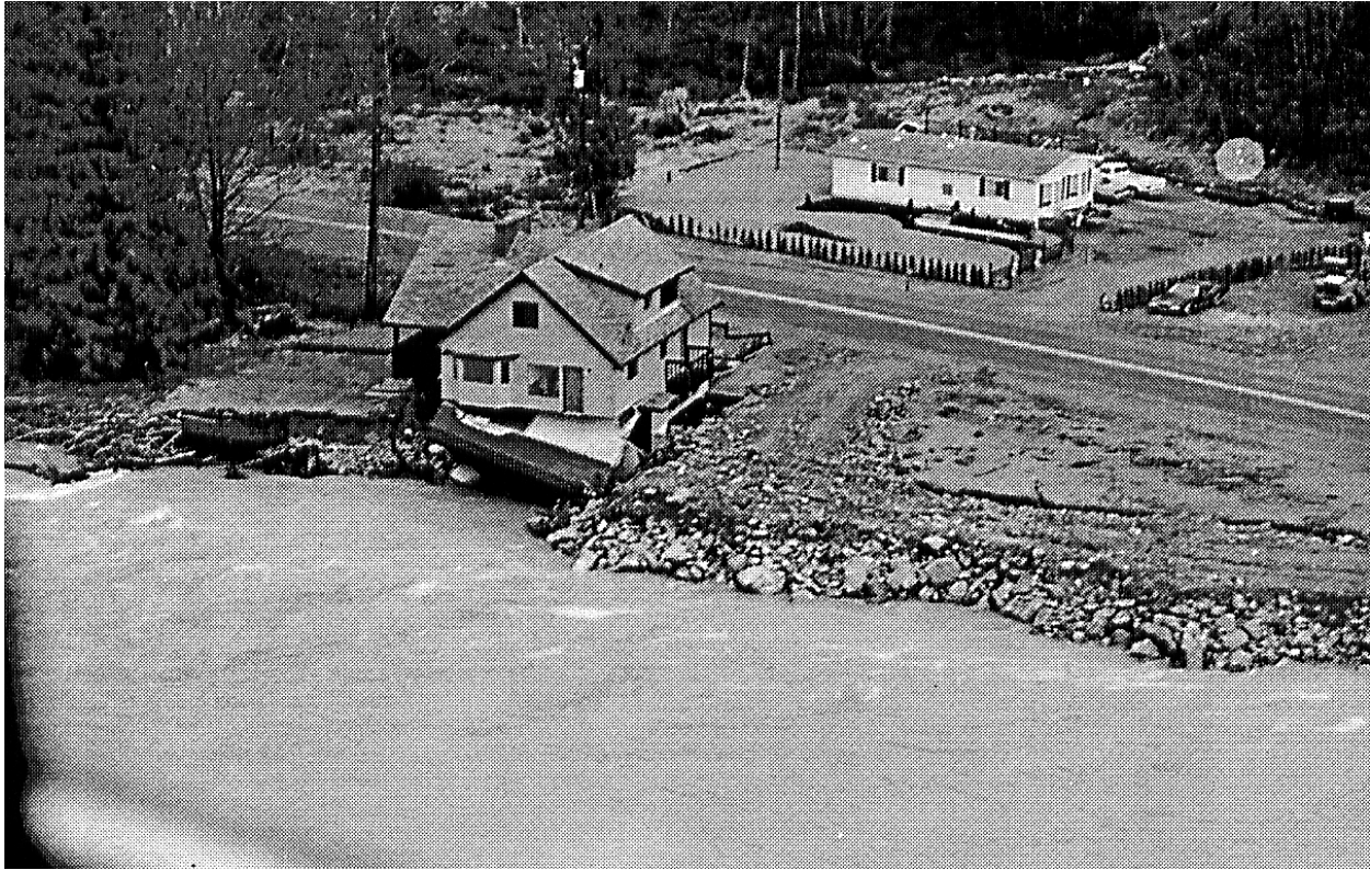
Figure 6-4: View of Riprap Placed Between Spurs to Reconstruct Bank Line
