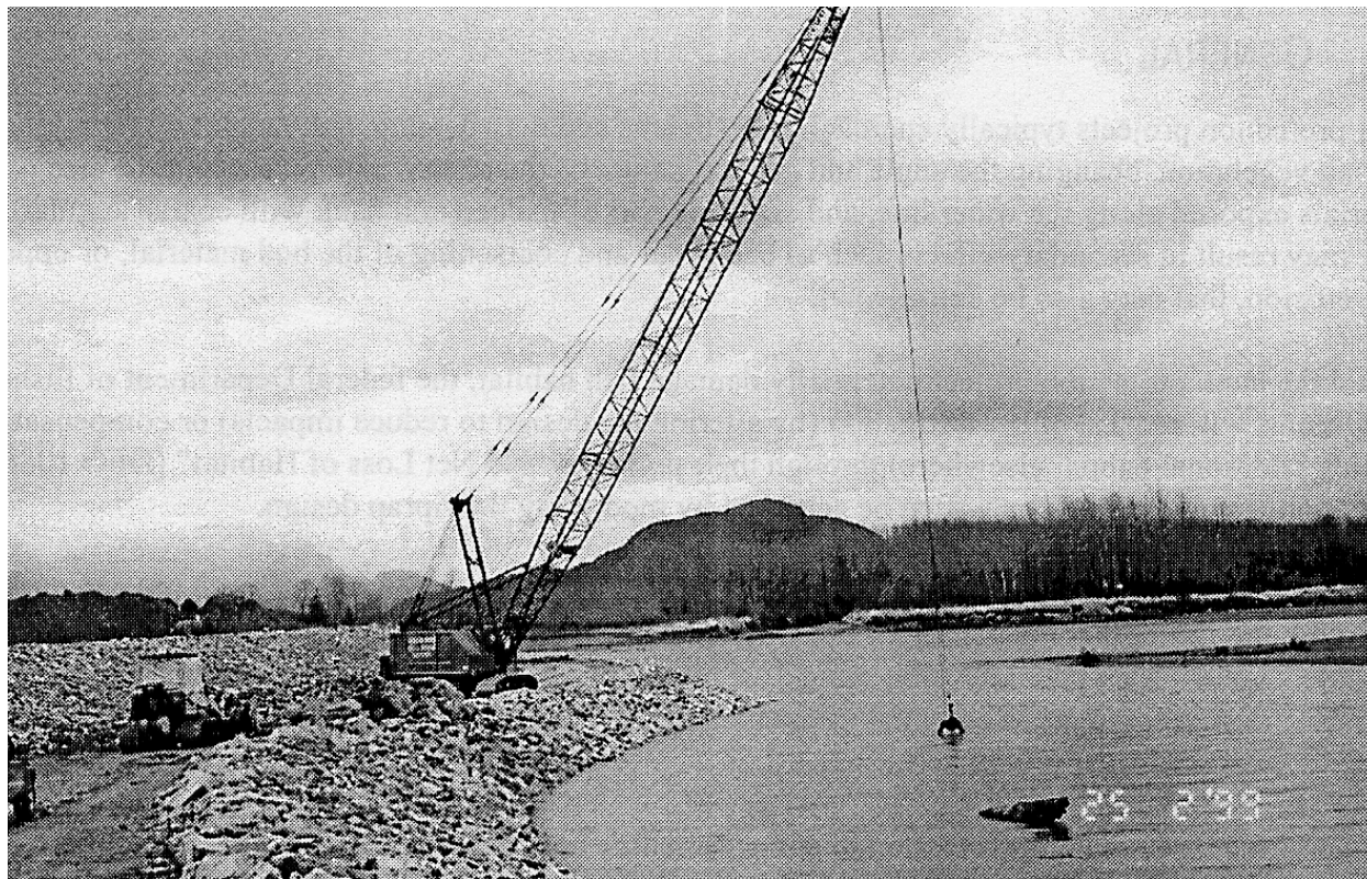
Figure 4-3: Placing of Toe Rock along Nicomen Island, Fraser River (1999)
