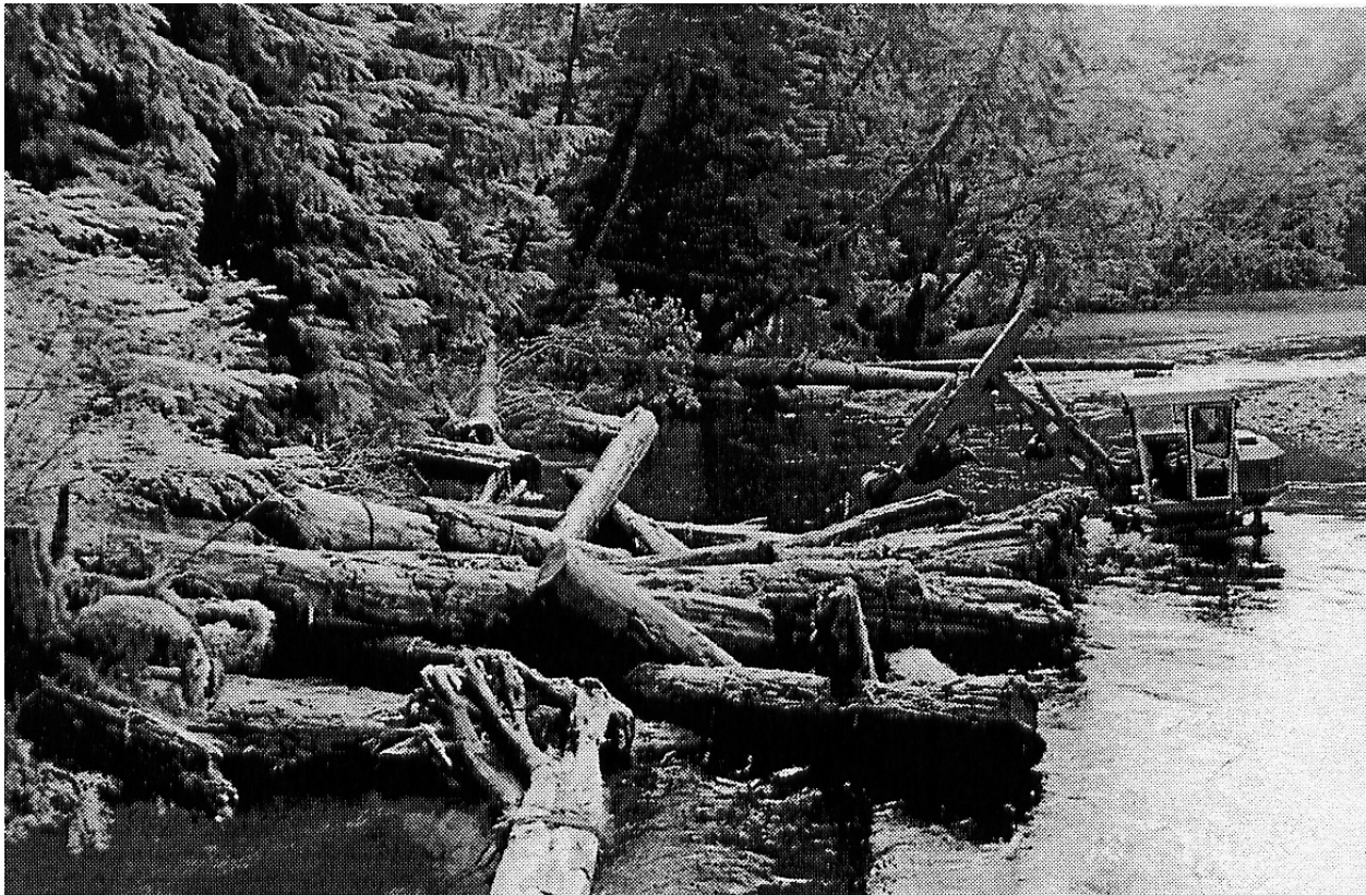
Figure 5-2: Construction of LWD Log Jam along the Mahatta River, Vancouver Island
